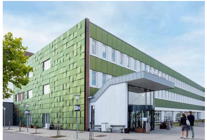
Bornholm Hospital was retrofit with exterior insulation and a custom solar rain screen.
