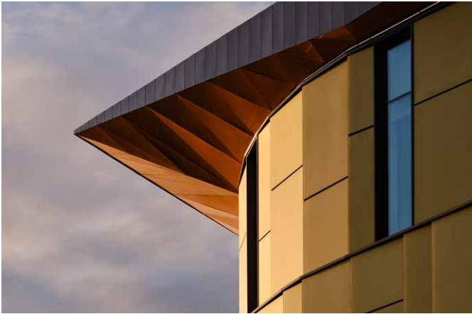
Red River College's Manitou a bi Bii daziigae building with varying panel sizes and a flowing facade, highlights the design freedom offered with a solar facade and the chameleon like nature of the color coating which provides a gentle and colourful addition to the campus.
