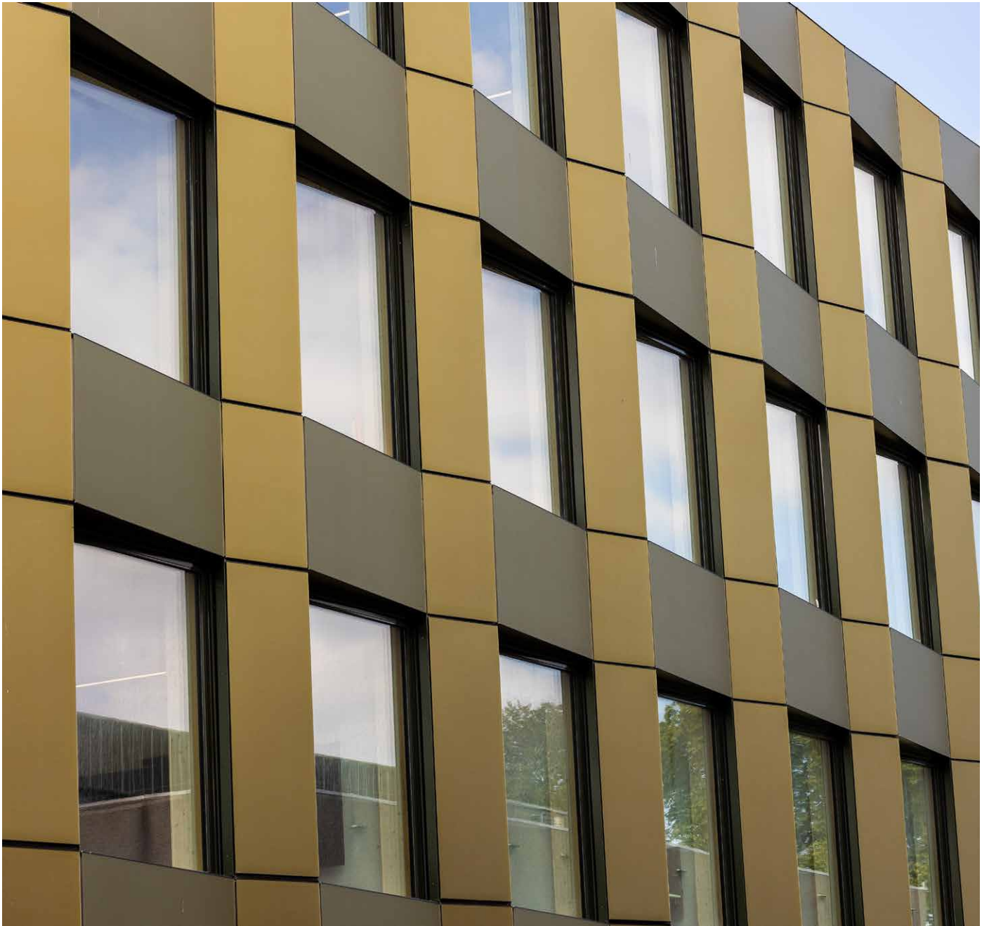
The deeply articulated facade of Breidablikk Gaarden in Norway offers passive shading and architectural depth.
